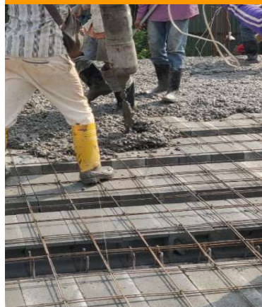
5 cm of concrete cast
