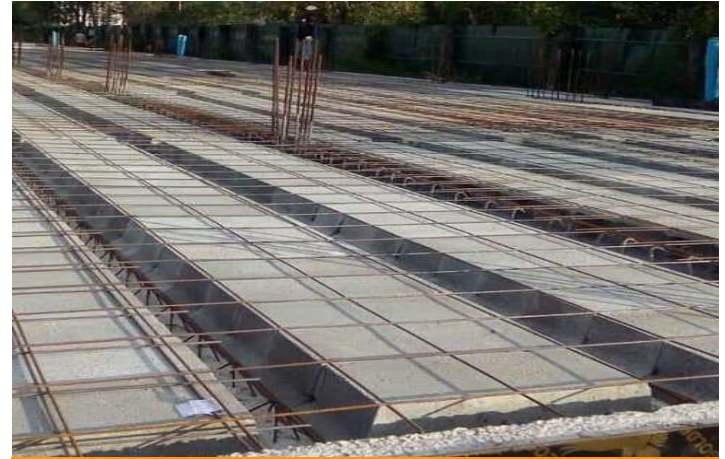
Welded steel mesh assembly
