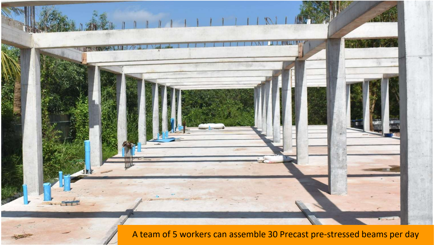
Precast pre-stressed beam retaining other beam
